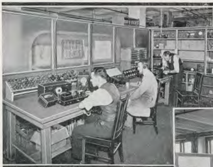
audio amplifier laboratory — In this section of the UTC laboratories, the development of transformers and amplifiers for public address and broadcast use is done.
